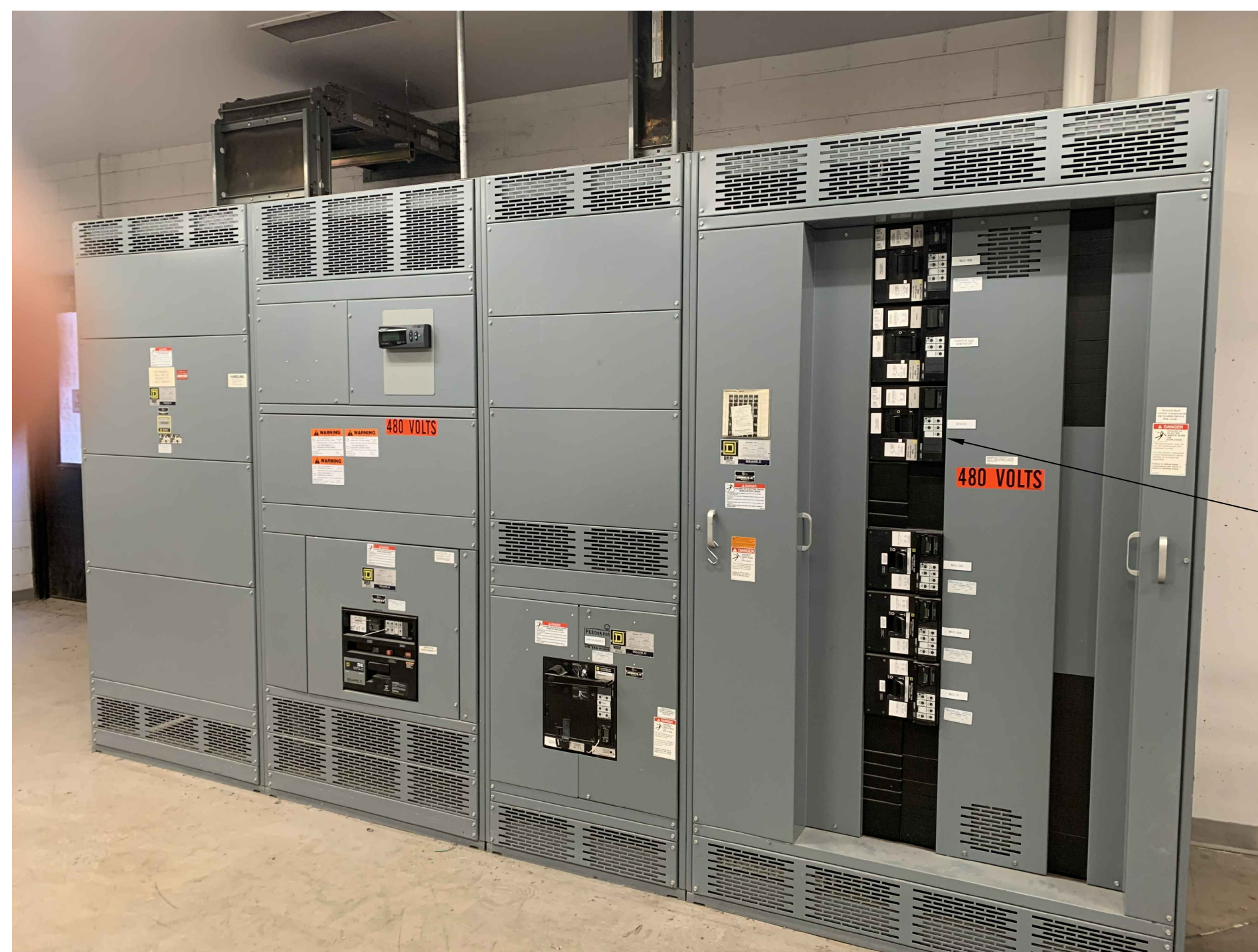
EXIST MAIN SWITCHBOARD SWBD-1 ELEVATION
