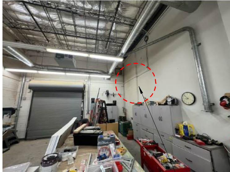
photo 10 NOTES: LOCATION OF NEW DOOR (DE2) - ENSURE NEW OPENING DOES NOT CONFLICT WITH ADJACENT CMU WALL.
