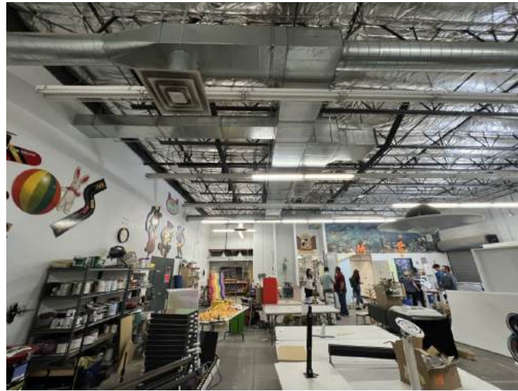
photo 2 NOTES: EXISTING ROOF INSULATION TO BE REMOVED AND SALVAGED. PREP FOR NEW PAINT AND FOR RE-INSTALLATION. EXISTING METAL JOISTS TO REMAIN.
