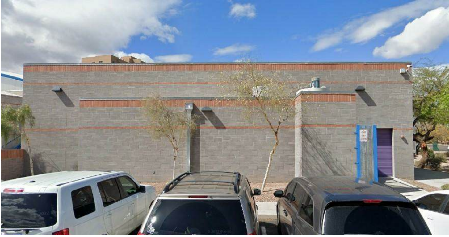
photo 2 NOTES: NEW OPENINGS IN EAST FACADE TO COURSE WITH EXISTING CMU MODULE.
