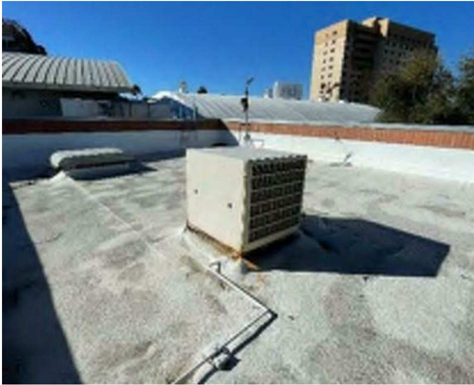
photo 3 NOTES: EXISTING CONDITIONS ON WAREHOUSE ROOF - EXISTING BUILT-UP ROOF SYSTEM OVER METAL DECK.
