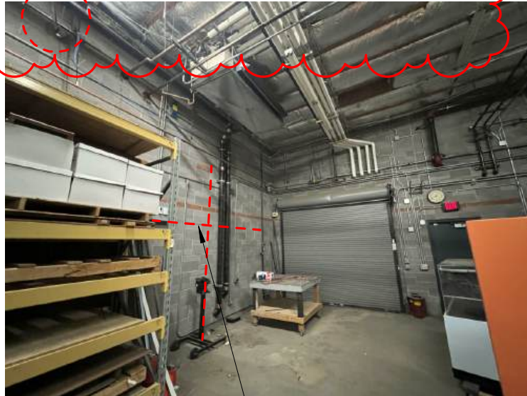
photo 11 NOTES: AREA OF SELECTIVE CMU DEMOLITION FOR INSTALLATION OF NEW DOOR. COORDINATE OPENING WITH EXISTING JOINT LINE - RELOCATE MINOR CONDUIT LINES, EQUIPMENT AS NEEDED FOR OPENING. REFER TO MEP + STRUCTURAL - NOTIFY ARCHITECT OF ANY DISCREPANCIES ON SITE FOR FURTHER DIRECTION.
