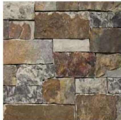
STONE VENEER FEATURE WALL
