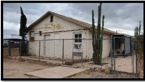
Figure 12b Milking barn Biggs Homestead 2305 N Mesa Drive. This was originally a milking barn for a dairy operated circa 1950, but since has been converted and upgraded.
