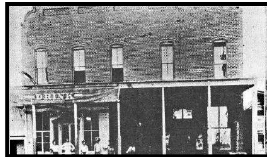
Figure 6a Pomeroy building in Mesa built of Lehi Red Brick 1891, Arizona Museum of Natural history (Mark, 2016)
