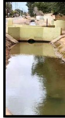
Open canal along Lehi Road
