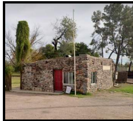
Figure 12a, Dairy Milking Barn on Mesa Drive built from river rock 2701 N Mesa Drive. It was used for both cow and goat Dairy farming.
