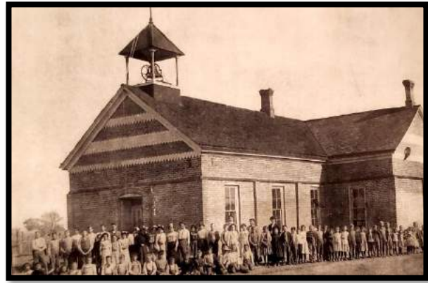
Figure 8, Brick Lehi Schoolhouse built with Lehi Red Bricks (Lisa A. Anderson 2008 Pg 18)
