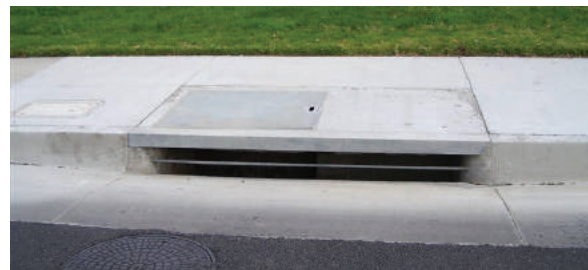
Figure 4-2 curb inlet style drain
