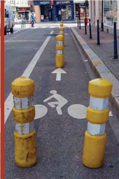
Inaccessible bike facilities often cause confusion to both cyclists and motorists.
