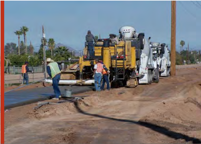
Consolidated Canal Phase 2 Construction
