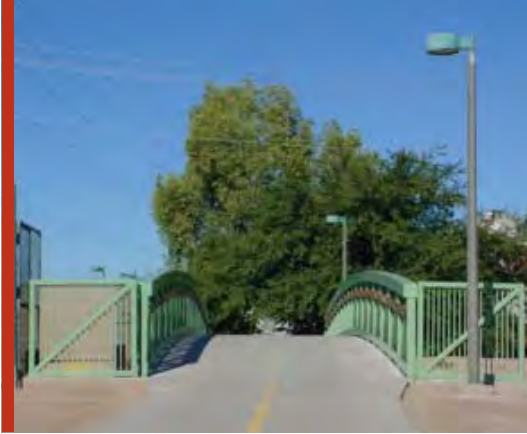
Eastern Canal Crossing at Pueblo Ave.
