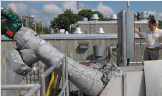
Heat Tracing and Blanket
