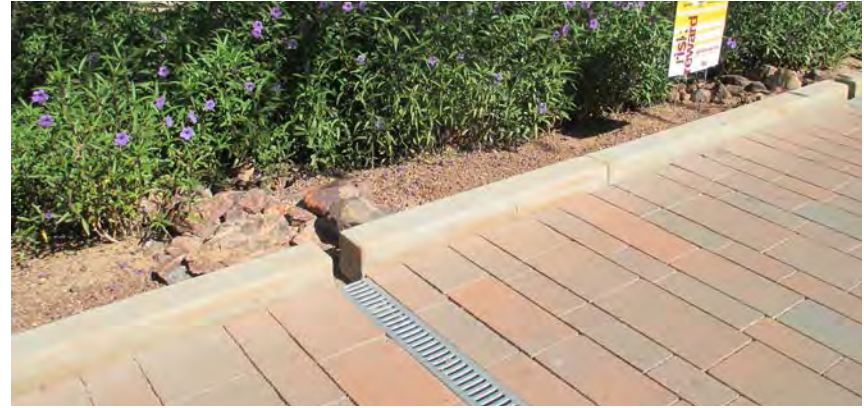
Grated curb cuts convey stormwater from pavement into planting areas.
