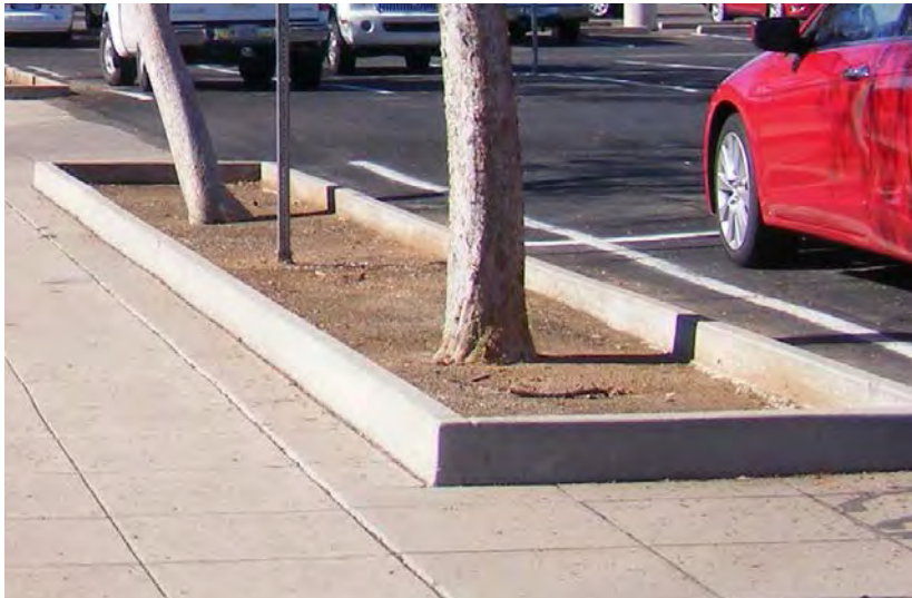
Existing Standard Curb
