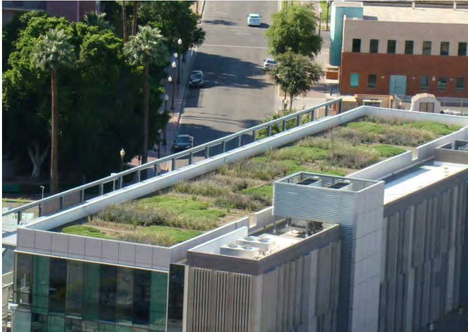
Green roof absorbs rainwater, provides insulation and creates a habitat for birds. It also helps to lower adjacent air temperature mitigating the heat island effect.
