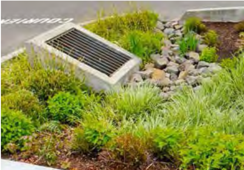
Sloped Grated Stormwater Sediment Capture and Bioretention
