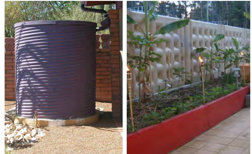
Cisterns can store rainwater to be re-used for future landscape irrigation.
