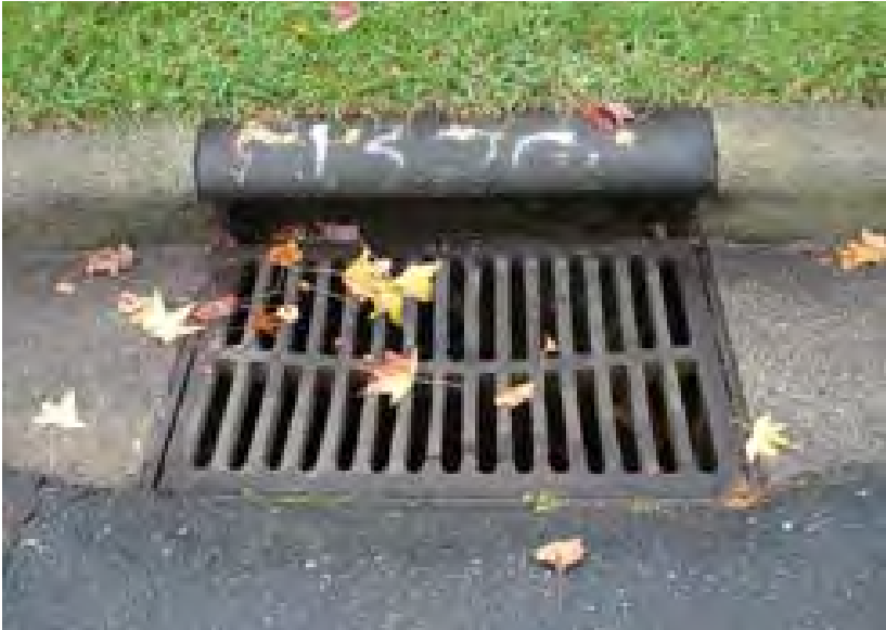
Existing Stormwater Catchment
