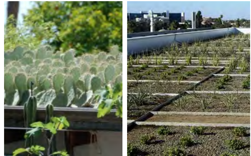
Green roofs store and utilize stormwater to reduce runoff from building sites.
