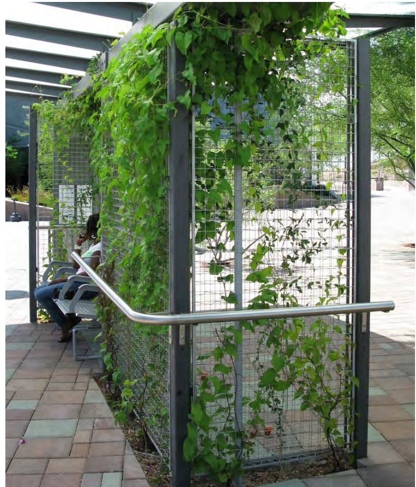
Shade structures at transit stations can harvest rainwater and use it to nourish a green wall.
