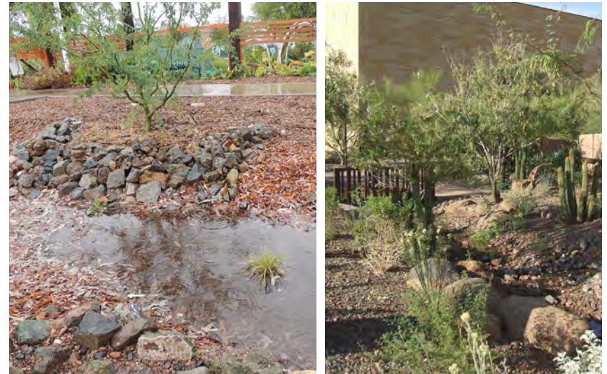
Vegetated swales accept stormwater for conveyance, storage and infiltration.
