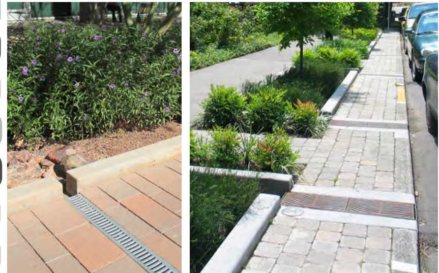
Grates allow stormwater to pass through while providing an accessible pedestrian route.
