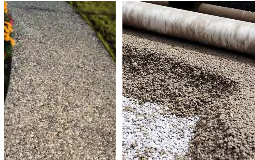
Porous concrete can reduce runoff sustaining in sidewalks and plaza areas.
