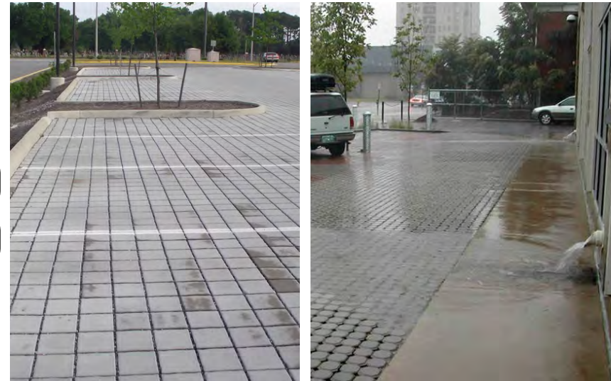
Permeable paving is an attractive way to provide runoff reduction in paving and pedestrian areas.
