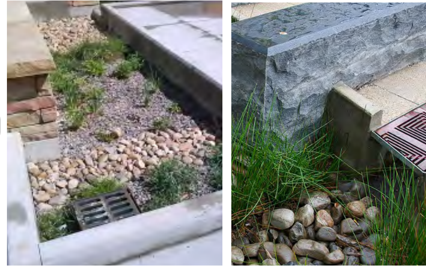
Bioretention cells fit into constrained urban site.
