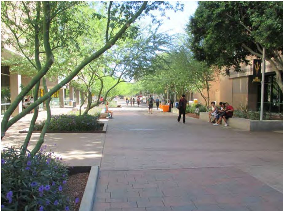
Porous pavers and permeable pavement at the pedestrian walkway allows infiltration and reduces off-site runoff.
