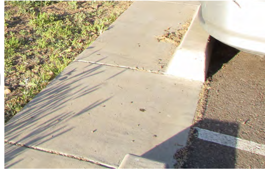
Wheelstops allow sheet drainage to pass into landscape areas.
