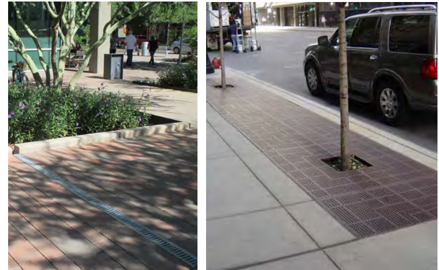
Bioretention planters provide stormwater storage and promote healthy growth of trees and plants.
