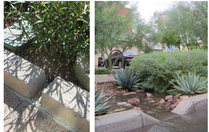
Curb cuts control stormwater flow from streets to LID facilities.
