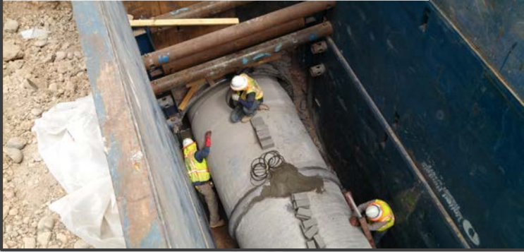
Val Vista Pipeline (Phases II & III)
