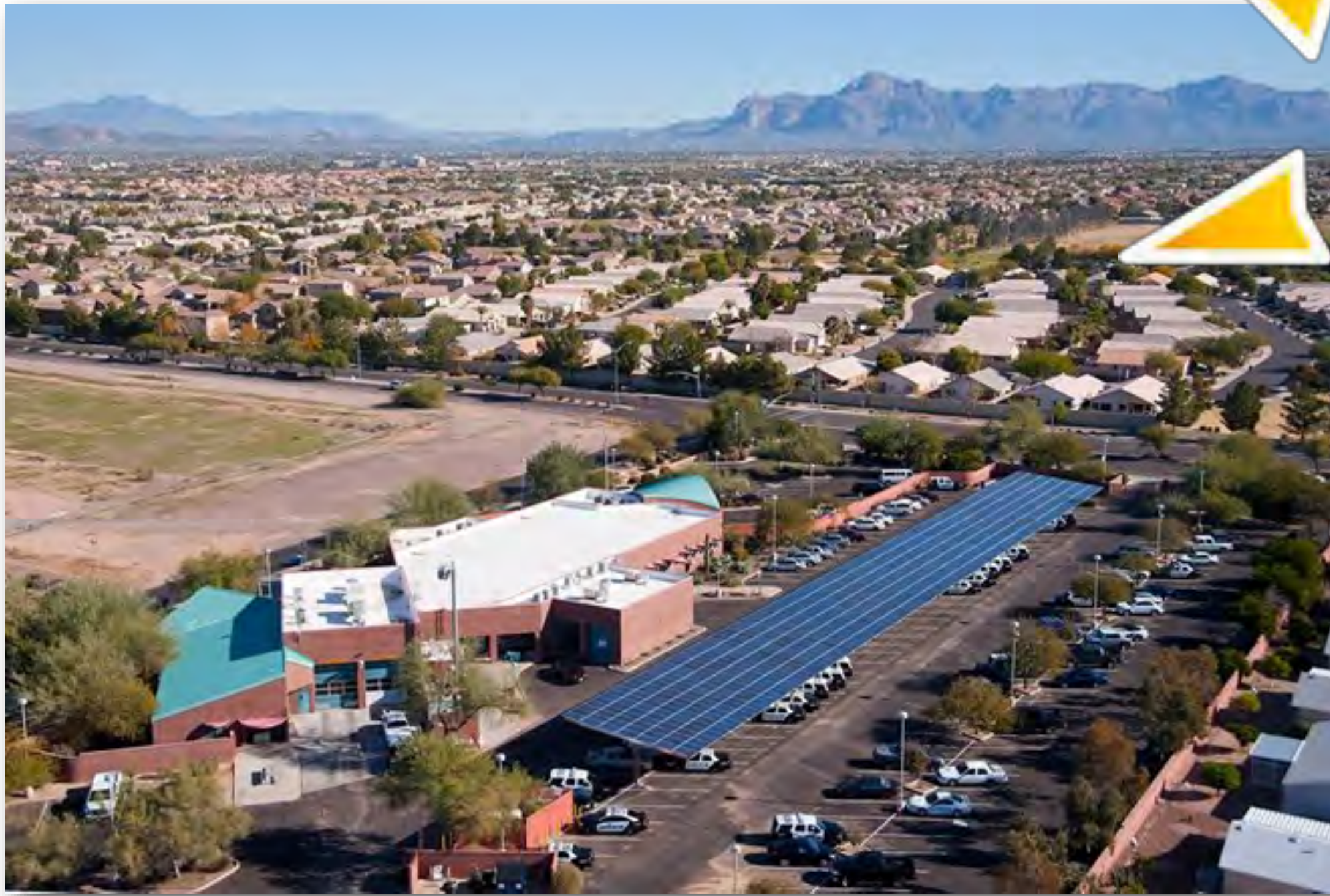
PD/FS 212 – 189 KW Photovoltaic Carport Mount
