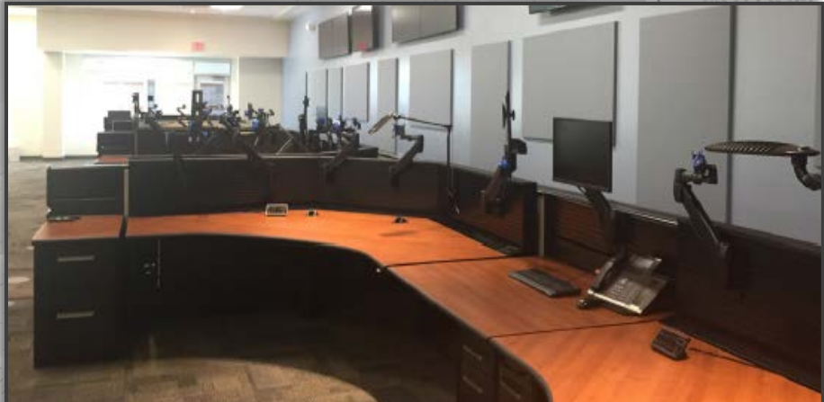
Fire & Medical Dispatch Center
