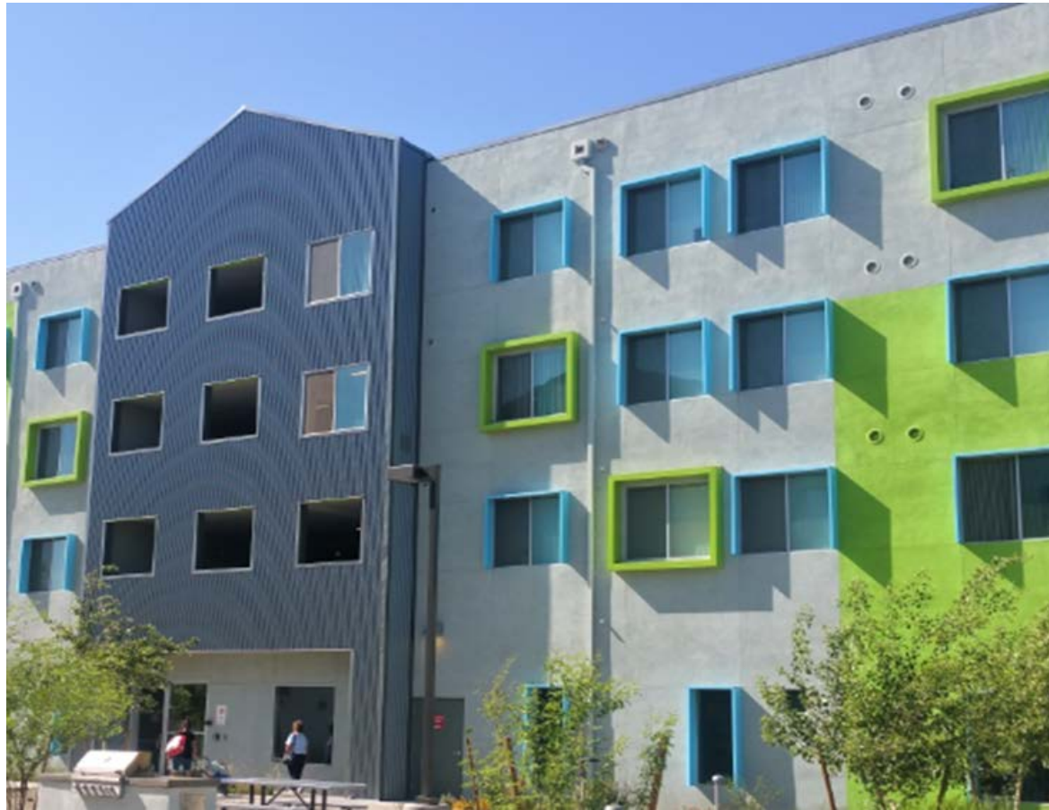
La Mesita Apartments
