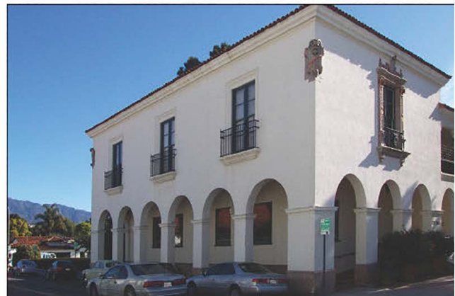
An example of an arcade encroaching the public ROW. The arcade provides the only means of circulation along the ROW.
