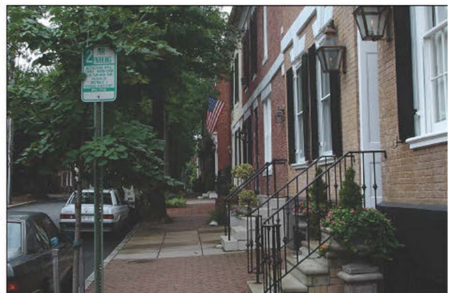
These stoops on townhouses with slightly recessed entries and a minimum setback allow the steps to engage the street.
