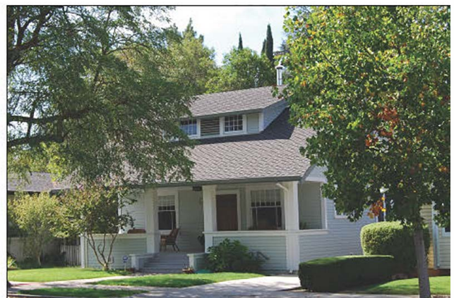
Projecting porch integrated into the overall massing
