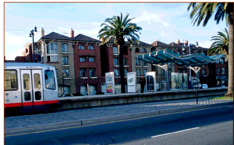
Embarcadero Light Rail Transit, San Francisco: Illustration of mixed-use moderate density development along light rail line.
