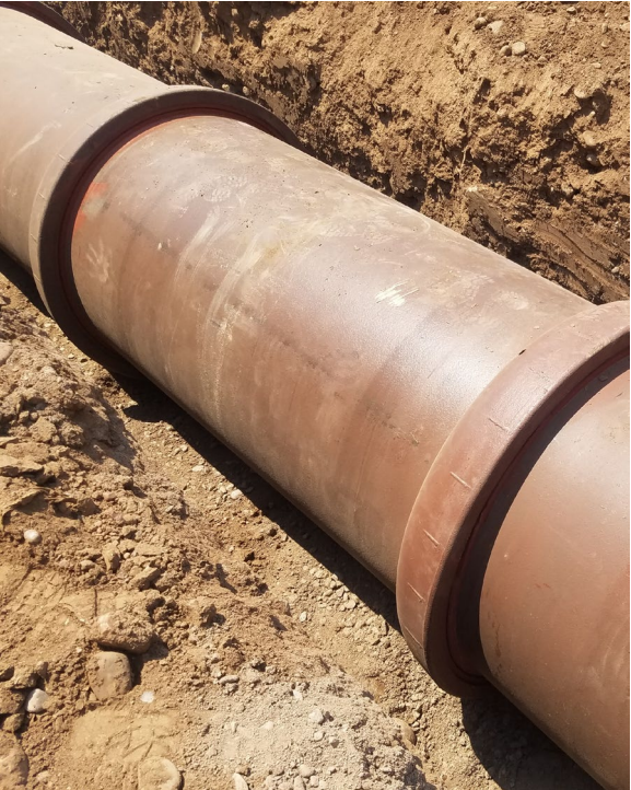
New Sewer Mains
