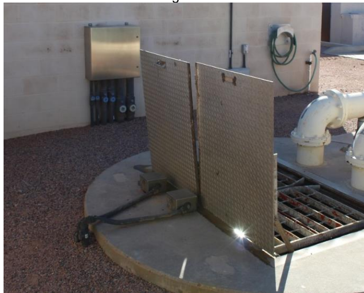
Figure 12 Existing Wet Well
